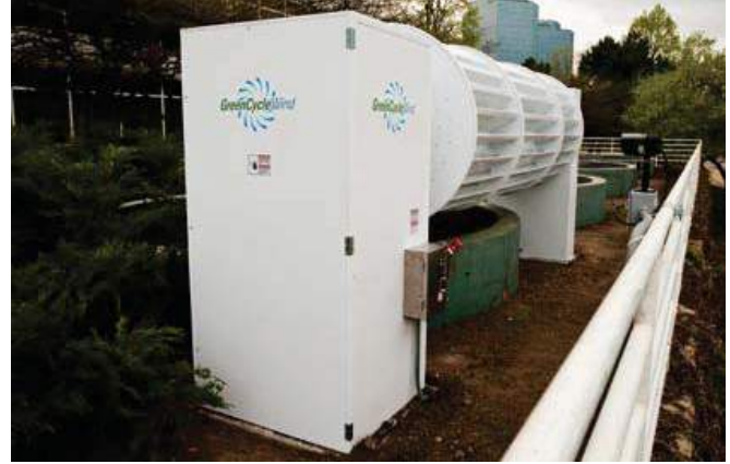
Fig. 1: Green Cycle Wind's turbine utilizes both natural and waste wind sources to reduce energy bill costs for companies.
